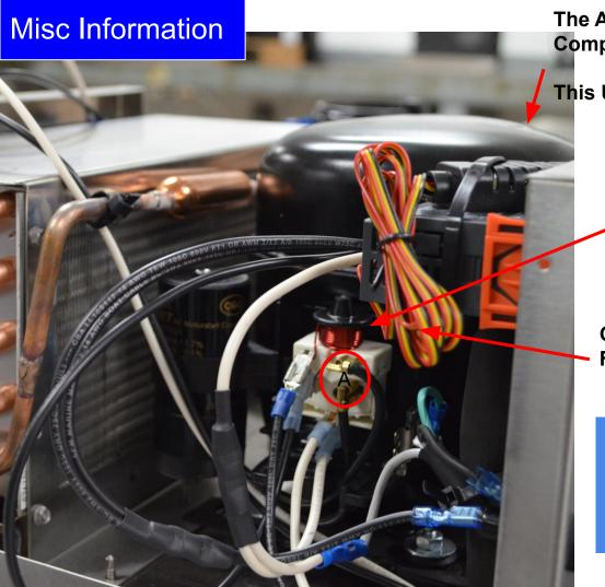
The Access Valve Is On The Other Side Of The Compressor.
