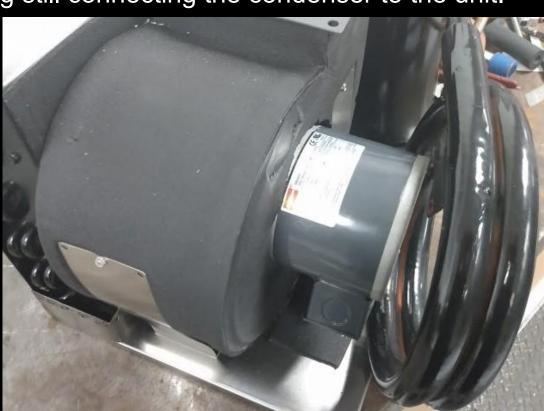
**Step 3** is to remove the screws attaching the top of the blower to the shroud. It will most likely be attached in one of the ways pictured below. Note a foam insulation will need to be scraped away enough to access these screws.
